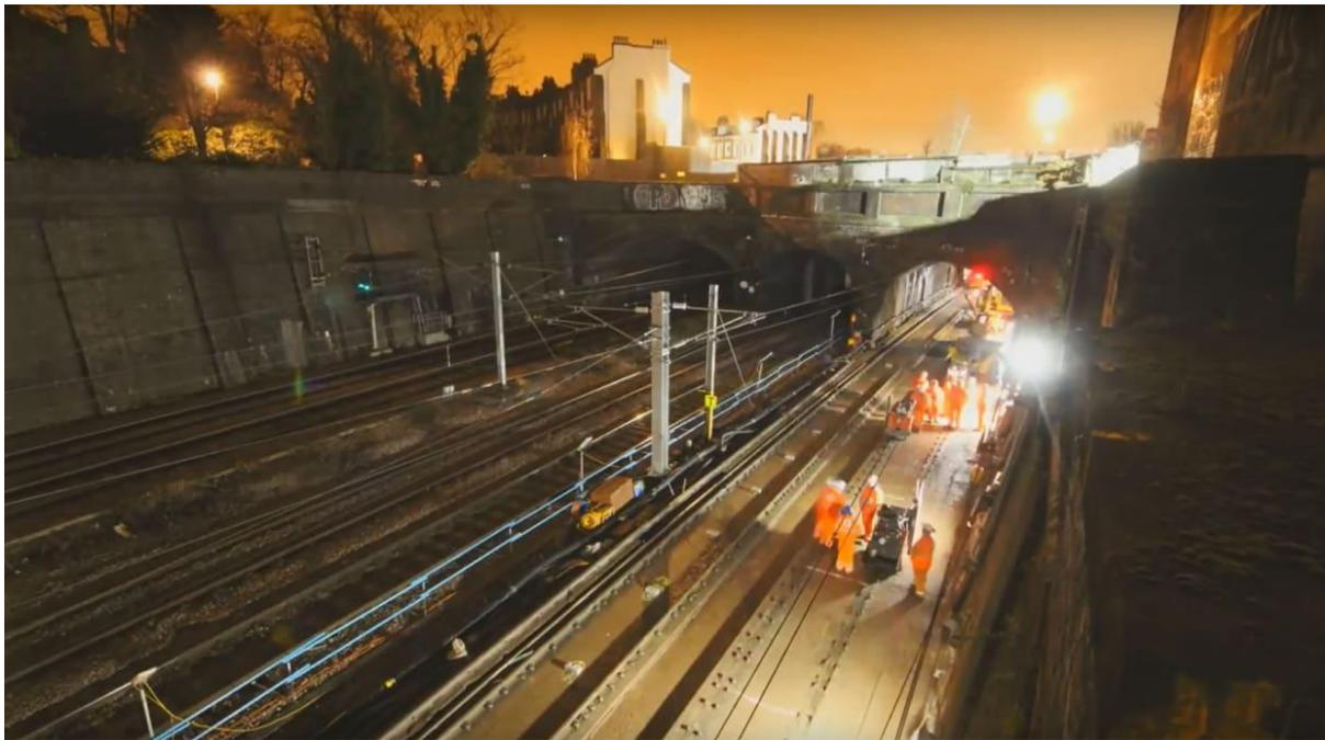
Between Christmas Day and Tuesday 4 January 2022, Network Rail engineers will work around the clock to remove the last section of slab track on the route, which was installed in 1979.
